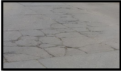
UM-25 (Prog. 1+173,867 a Prog. 1+197,746) Losas dividida
