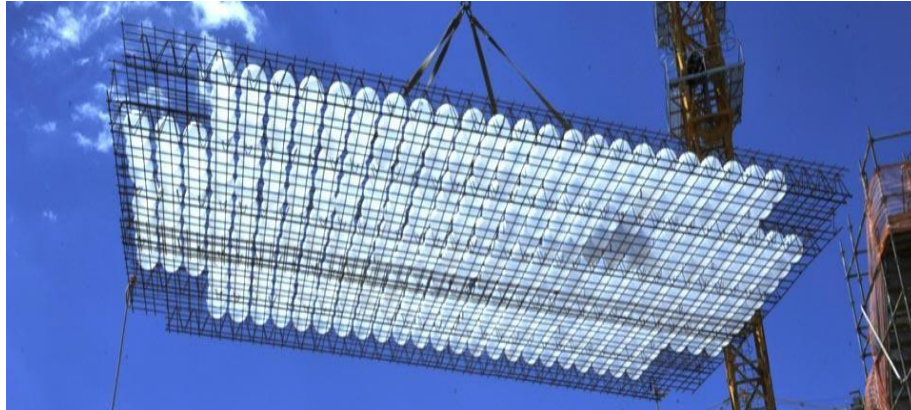
Figura 2.11 Losas Bubble deck (Reinforcement modules). [4]
