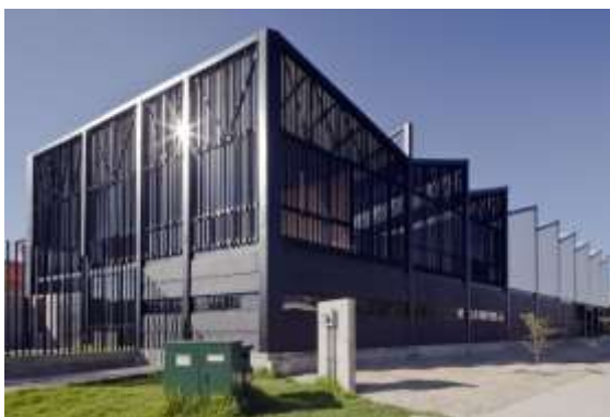
FIGURA 6: LEVERING TRADE - ARQUITECTURA INDUSTRIAL
