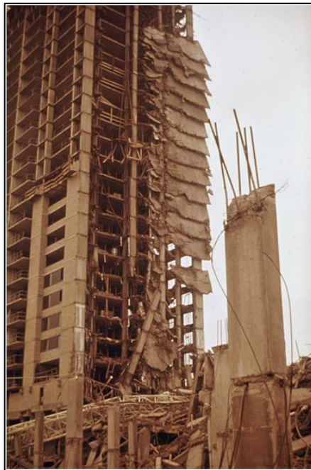
Fig.1.1 Colapso del edificio Skyline Plaza Apartment Building
