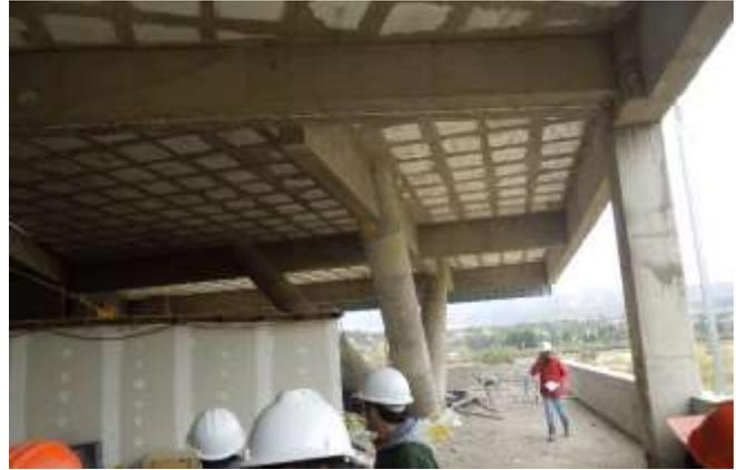
MUROS EXTERIORES CON PLACAS DE YESO DE 12 MIM LXA =2,40 X 1,10
